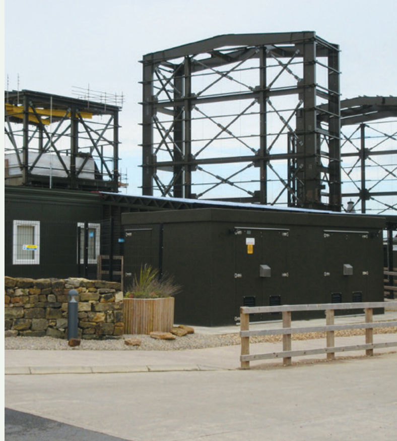
On hold: Lockwood Beck tunnel access March 2020
