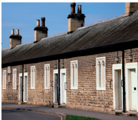
Lady Lumley's Almshouses in Thornton
