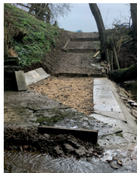
Horse-friendly ramp under construction
